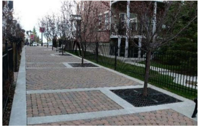
Figure 4.65: Pervious pavers with tree wells
