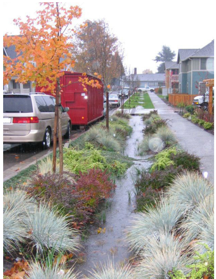
Figure 4.66: Bioswale filters stormwater
