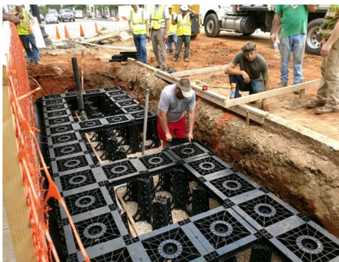
Figure 4.64: Tree wells with Soil Cells
