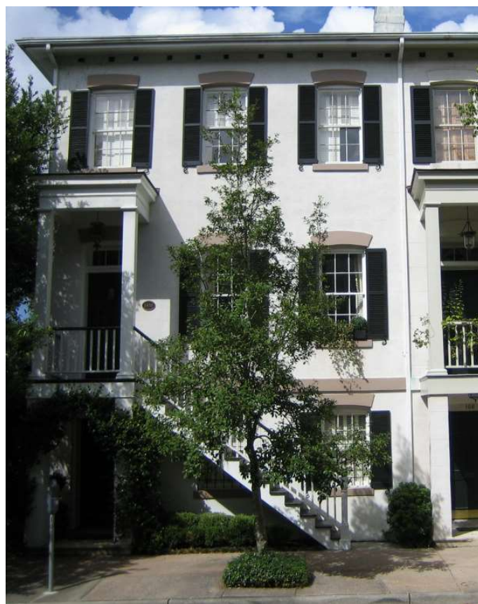
Figure 5-18: An at-grade entrance, and an exterior stair leading to the entrance of the unit above
