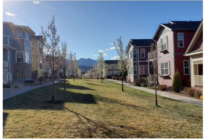
Houses front onto a Green Street with garages and driveways accessed from a Rear Alley.
