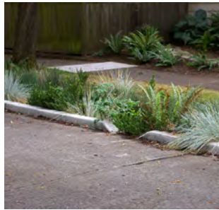
Planting Strip Trench
