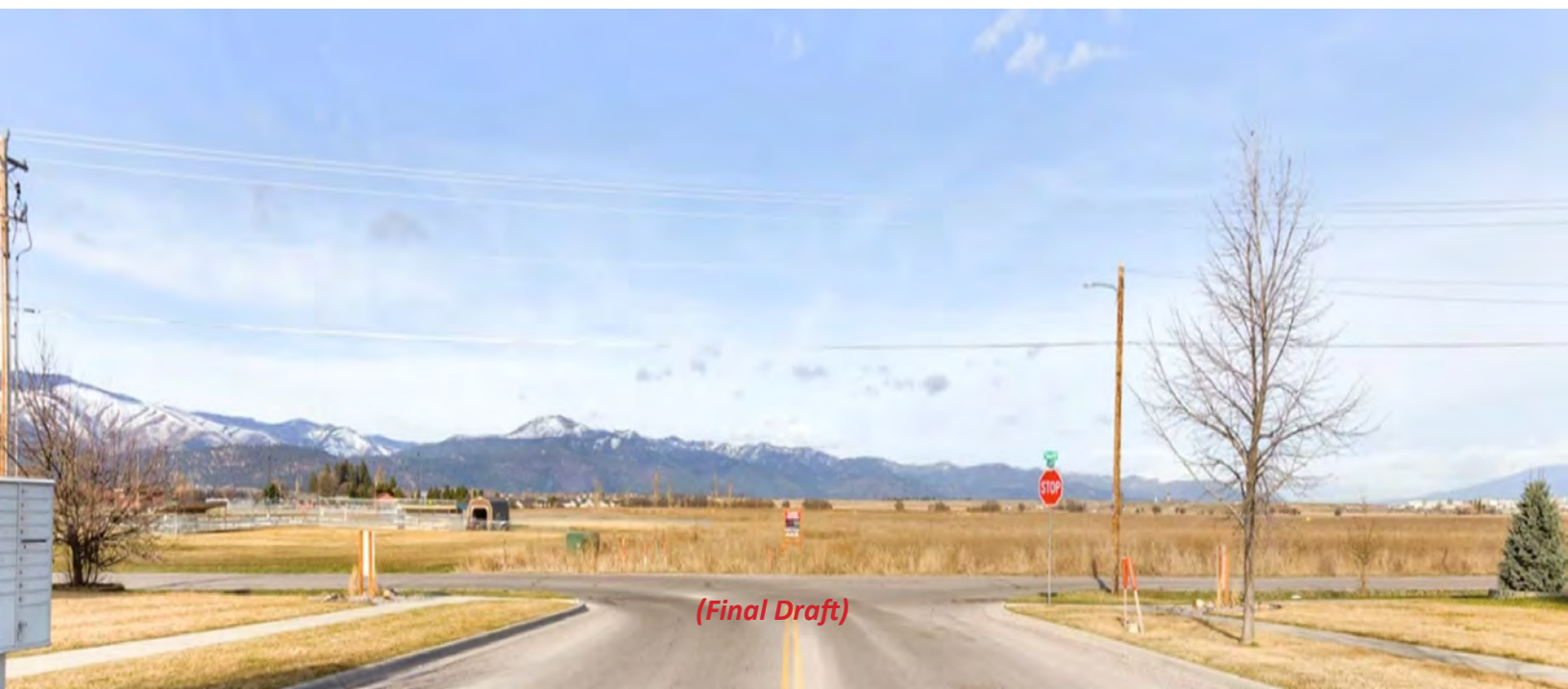
Existing road in the Mullan Area
