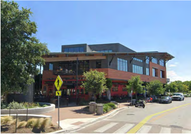
Office and research buildings create a walkable urban form.
