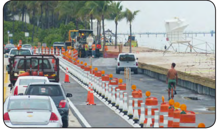
After Hurricane Sandy A1A in Ft. Lauderdale was washed away. The new road is higher & lined with walls.
