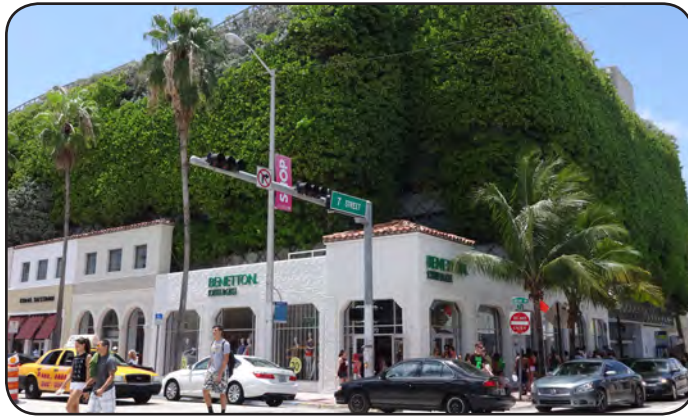
Collins Avenue, Miami Beach, Miami-Dade County
