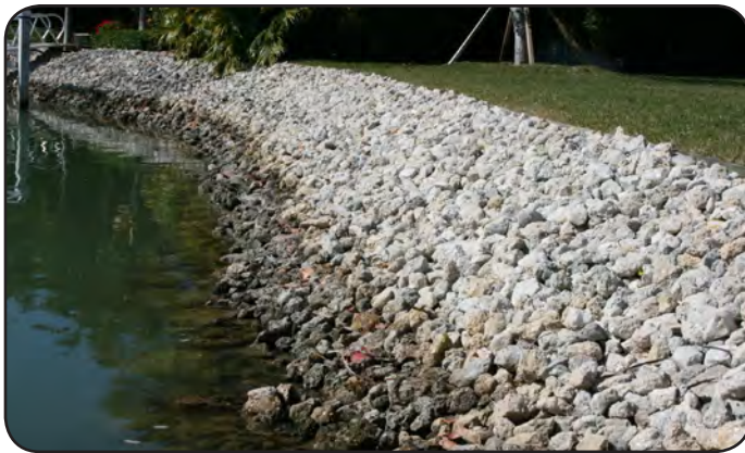
Rip rap along a shoreline
