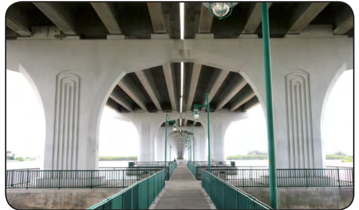
Barber Bridge, Vero Beach, Indian River County
