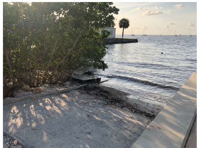
Manual boat launch ramp in Gilchrist Park, Punta Gorda
