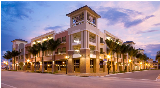
Herald Court Centre; Photo credit: City of Punta Gorda
