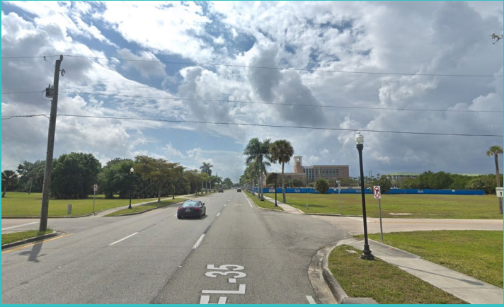
Existing conditions - Marion Ave
