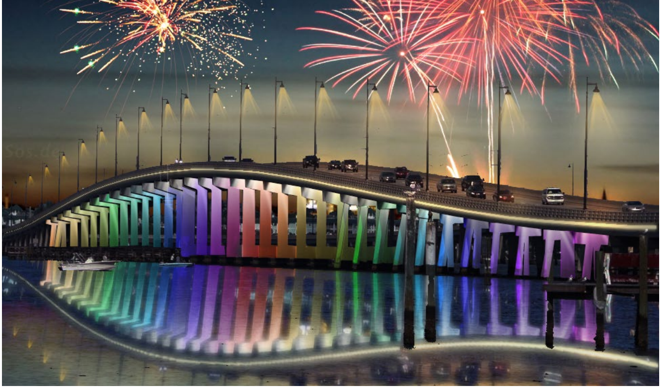
Gilchrist Bridge Lit Up with Rainbow LED Lighting for a Special Event
