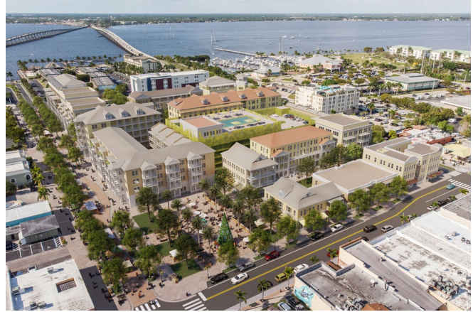
City Market Place Development Option 2: Higher intensity mixed-use development with new public spaces
