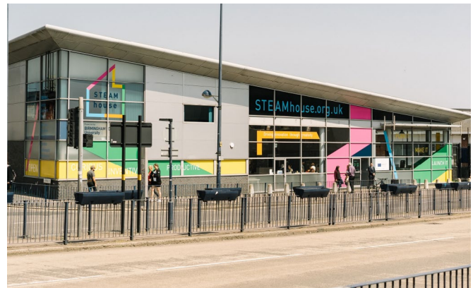
STEAMhouse fabrication center, part of Birmingham City University in Birmingham, UK
