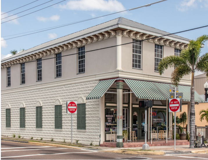
264 W Marion Ave; Commercial Vernacular Style 1909
