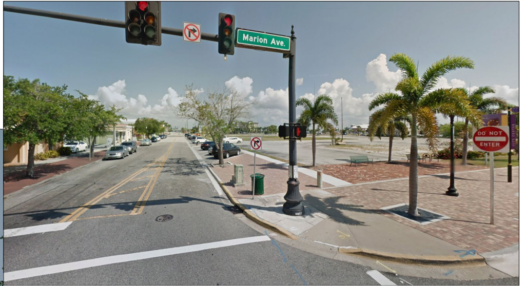
Taylor St and Marion Ave - Existing Condition
