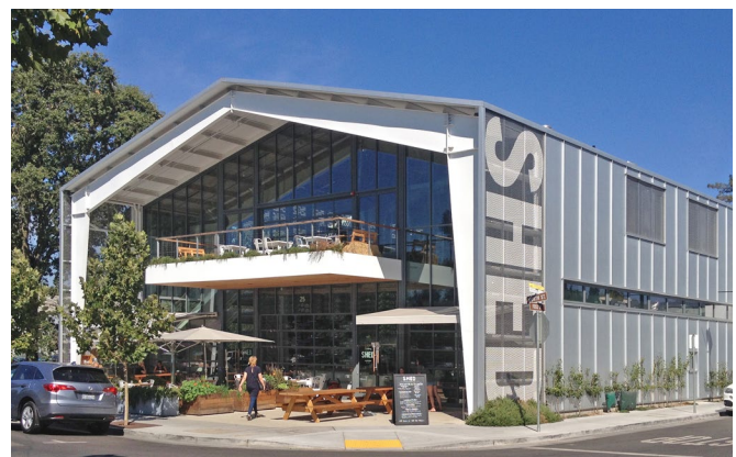
Prefabricated shed building, designed as a flexible space that could accommodate a market hall, small brewery, and events (Lincoln Lighthill Architect)
