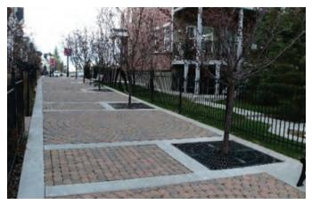
Figure 2.23: Pervious pavers with tree wells
