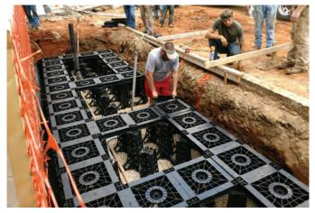
Figure 2.22: Tree wells with Soil Cells
