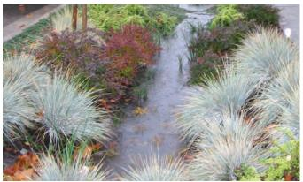
Figure 2.24: Bioswale filters stormwater
