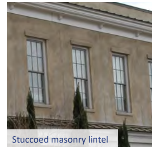
Stuccoed masonry lintel
