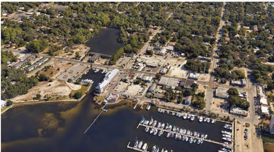
Below: Existing conditions
