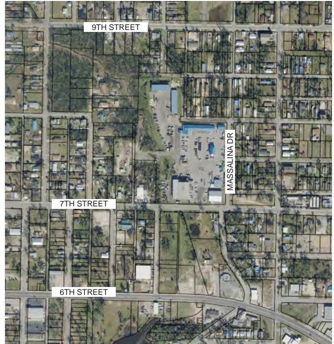
Existing conditions; although portions of the flow have been altered, the path of water to Massalina Bayou is evident in the aerial photo.
