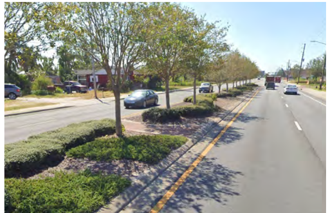
Above: Example of existing long median on MLK Jr. Blvd.
