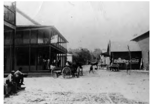
Tarpon Street and 3rd Street
