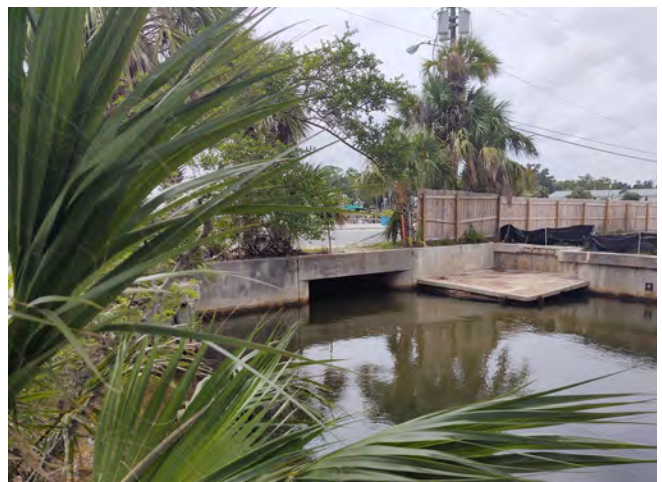
Above: Existing Marina entry
