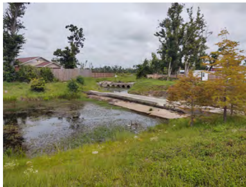
Above, top: Existing drainage channel at Lincoln Drive & 15th Street
