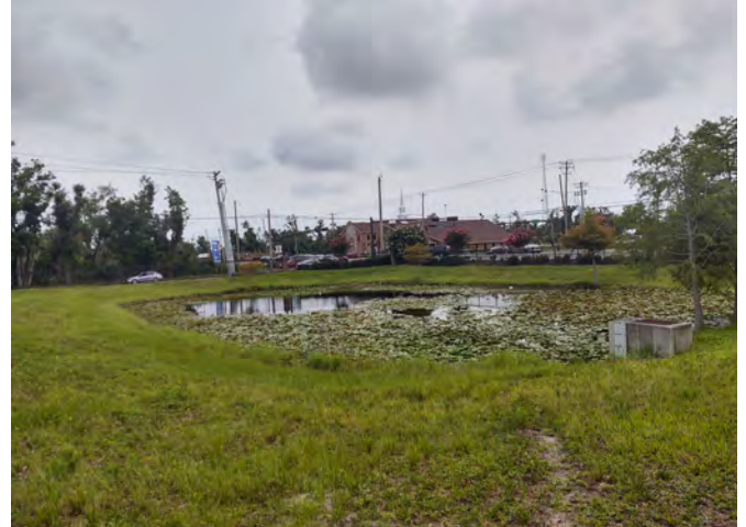
Example of engineered channels and ponds needing restoration and naturalization at MLK Boulevard & E 11th Street.
