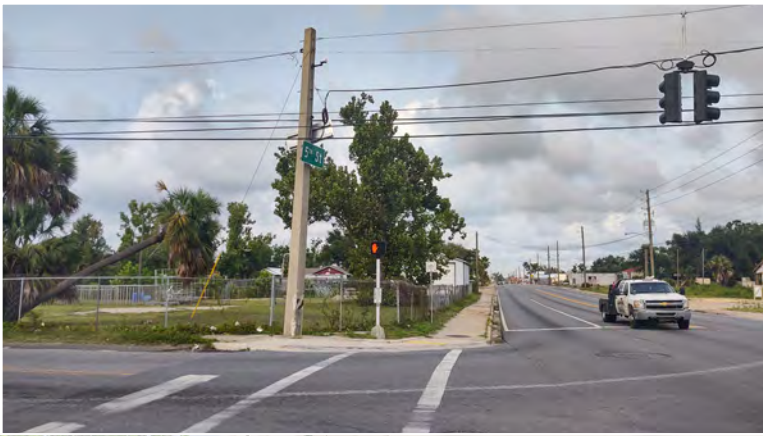
Left: Existing conditions of Business 98 and Sherman Avenue.
