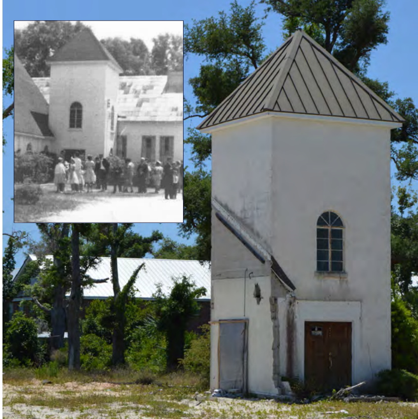
Trinity United Methodist Church - 1958 historical photo shown in inset and remaining structure, post-Hurricane Michael
