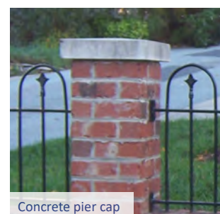
Concrete pier cap
